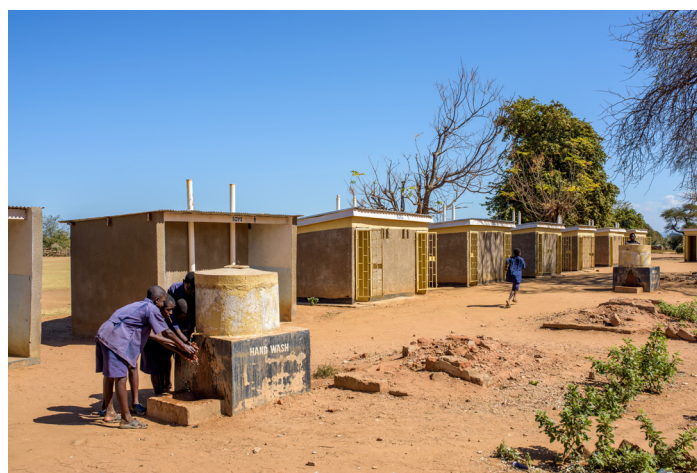
Latrines and hand-wash stations built by World Vision Zambia at Malima Primary School, Sinazongwe Area Programme
